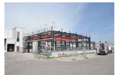
Construction site June 2014
