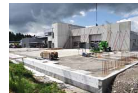
Construction site middle of May
