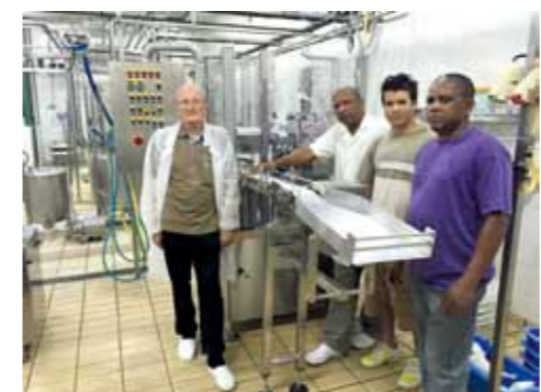
Photo below (from left to right): After completion of the installation and commissioning of the HITTPAC AKH-019R through Beat Beck, José Pedro R. Andrade, technical director, and the machine operators Kenny and Carlos
