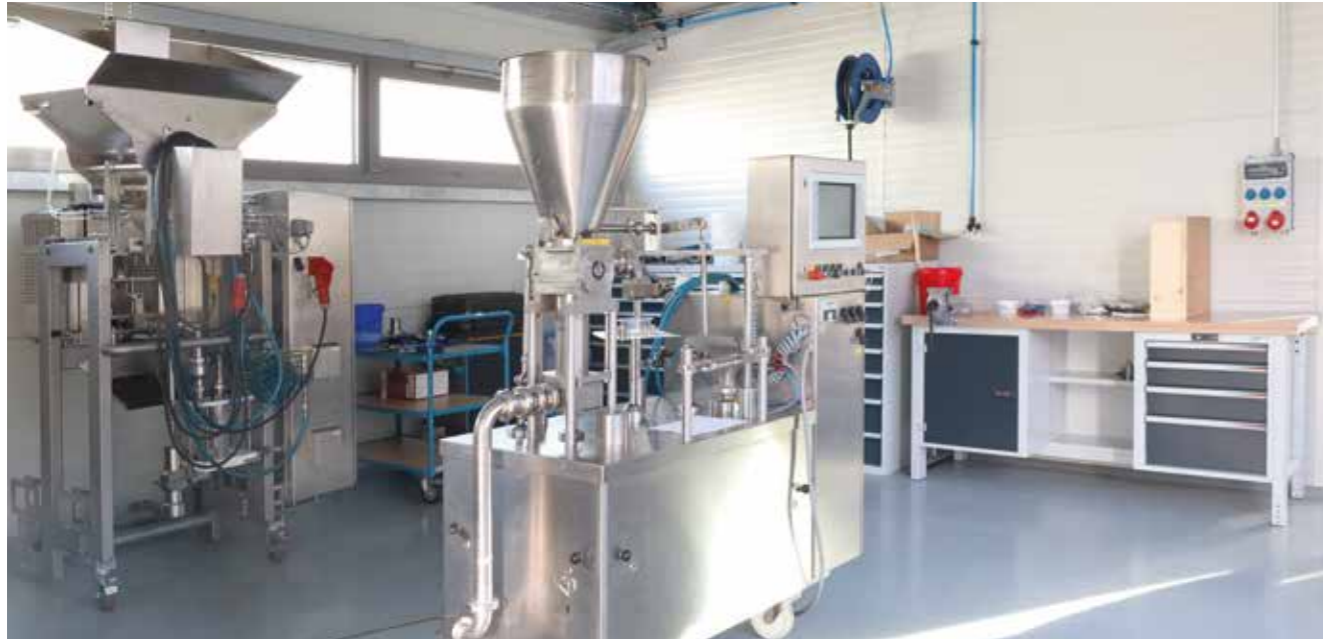
View into one of the laboratories of the new GRUNWALD development centre for filling trials and tests of a wide variety of products
