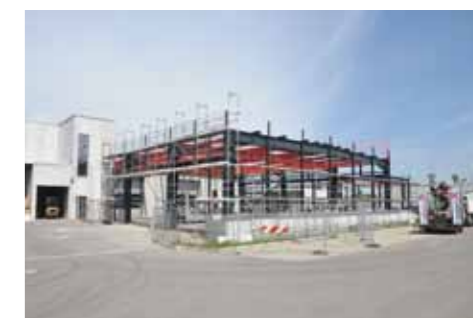
Construction site June 2014
