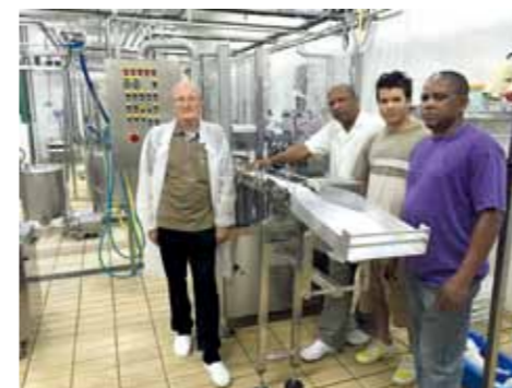
Photo below (from left to right): After completion of the installation and commissioning of the HITTPAC AKH-019R through Beat Beck, José Pedro R. Andrade, technical director, and the machine operators Kenny and Carlos
